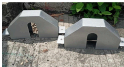
Figure 3.16 Bearing covers
